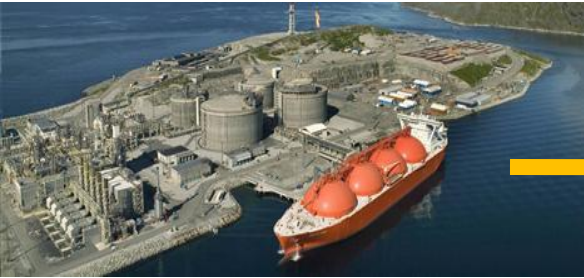
Base load plant
