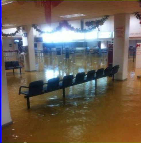
Hewanerra Airport flooded during Christmas Eve 2013 trough
