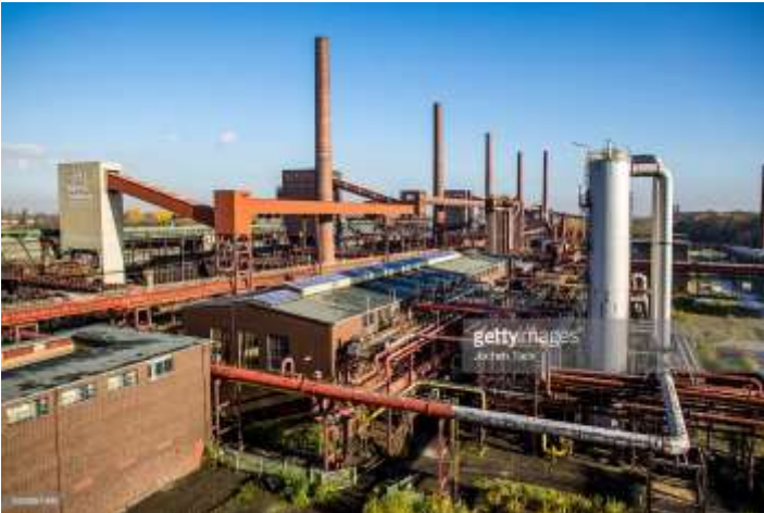
Construction of Coking Plants near Mongolian Coal Mines
