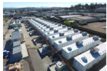
AES & SIEMENS – Escondido, California, EEUU 30 MW/ 120 MW/h Capacity: 20.000 homes for about 4 hours
