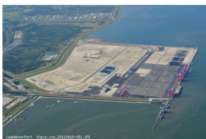
Jade Weser, Wilhelmshaven, opened in 2012 as the 1 st deep-water container terminal in Germany, which has a natural depth of 18m.
