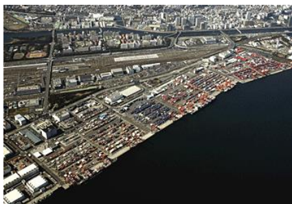
Ohi Terminal, Tokyo, opened in 1970s, was reconstructed to deepen its water-depth alongside from 13m to 15m.
