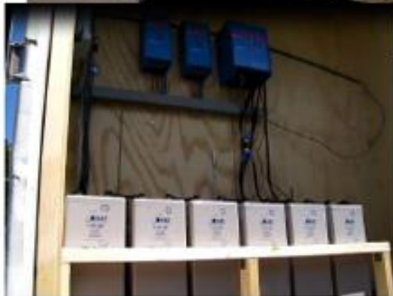
Batteries and inverter system
