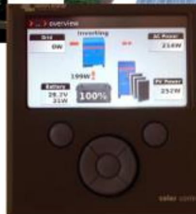
Solar monitoring system (also remote monitoring)
