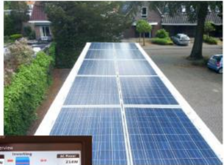
Solar panels mounted on roof
