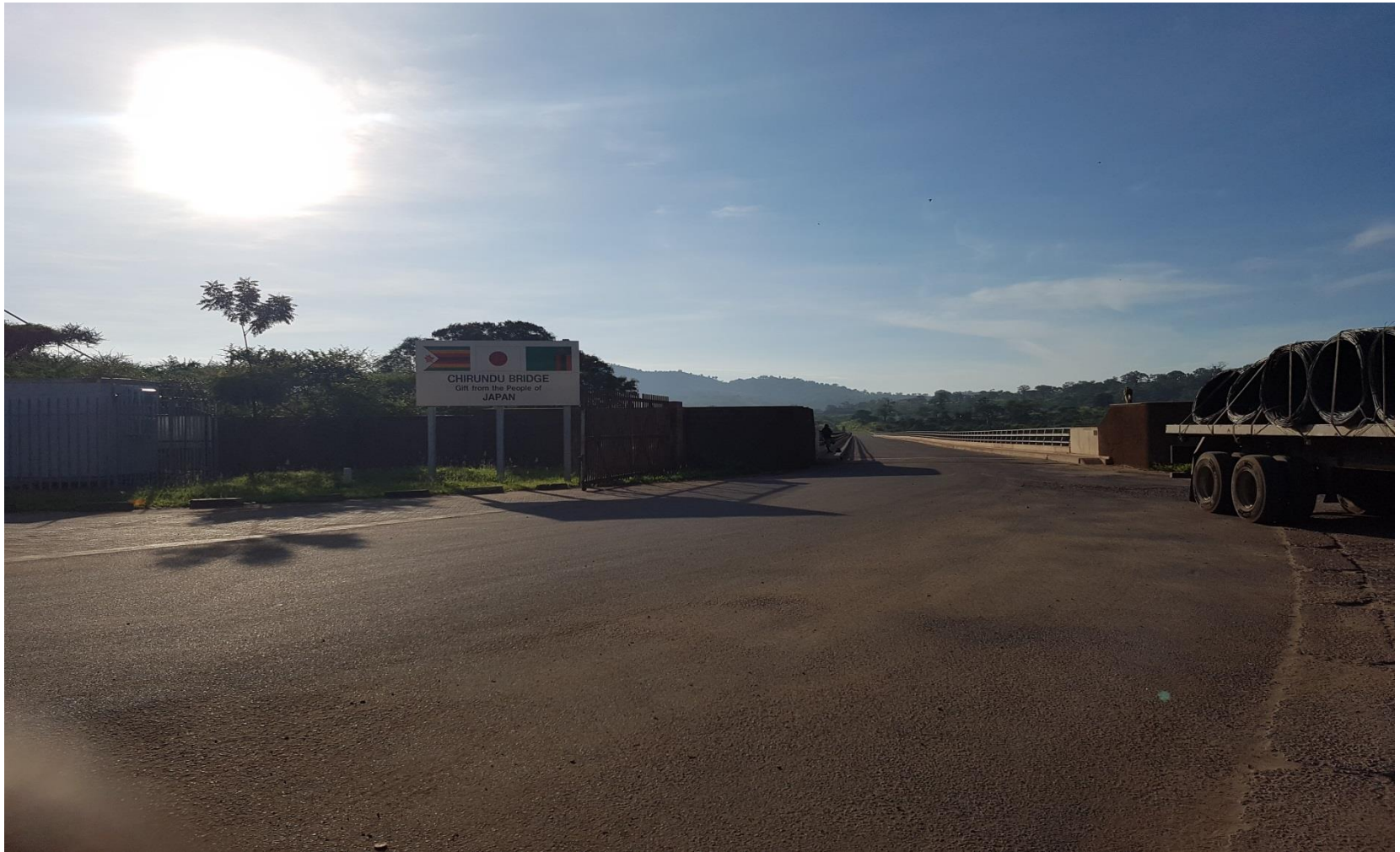
New Chirundu bridge connecting the two OSBP facilities
