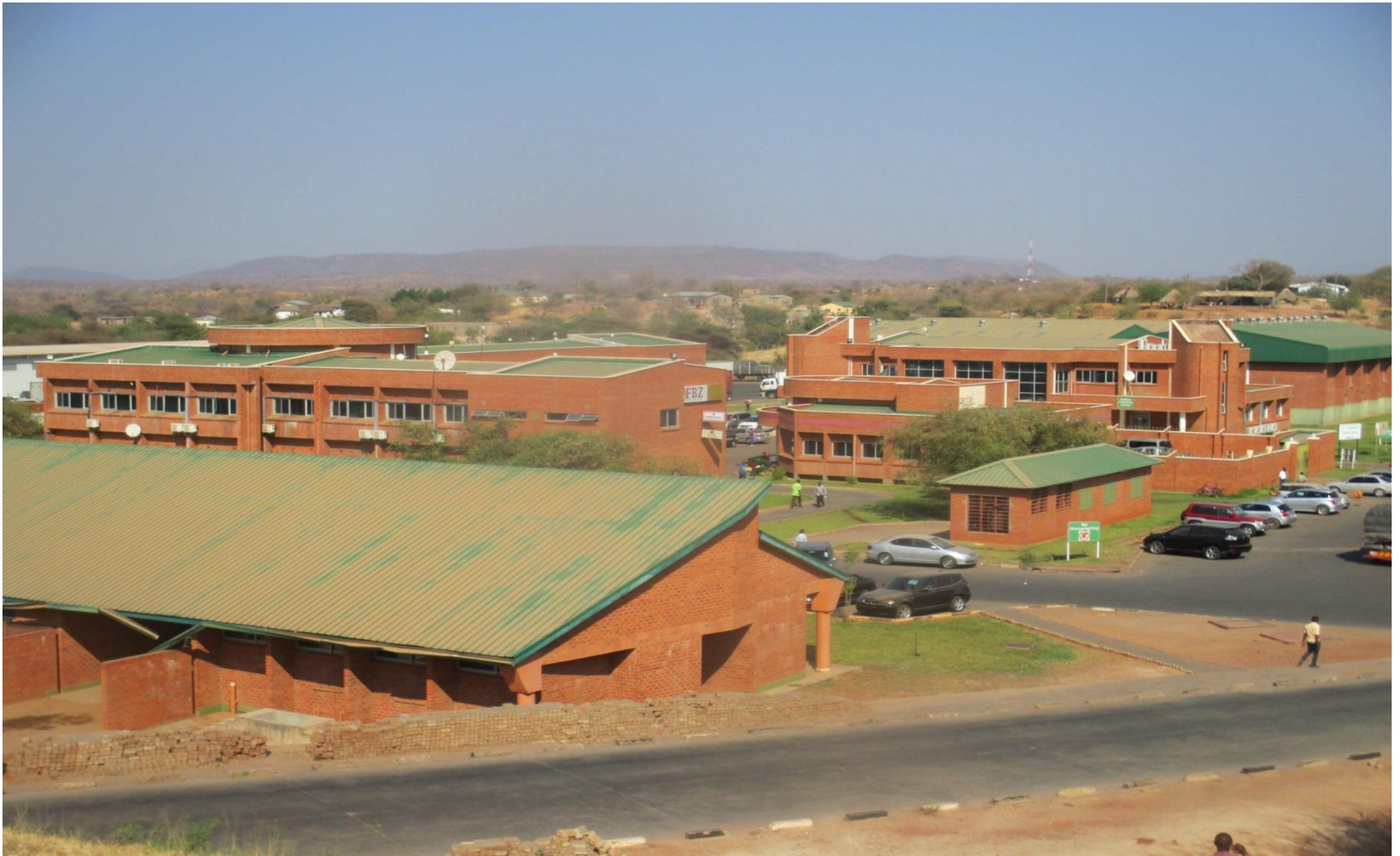
New Chirundu OSBP Border facility; Zambian side
