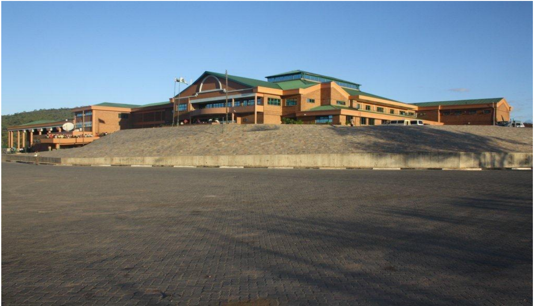
New Chirundu OSBP Border facility; Zimbabwean side
