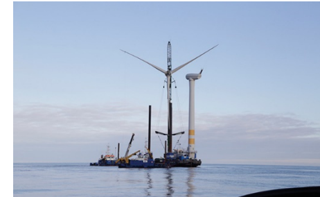
First Decommissioning of an Offshore Wind Farm
