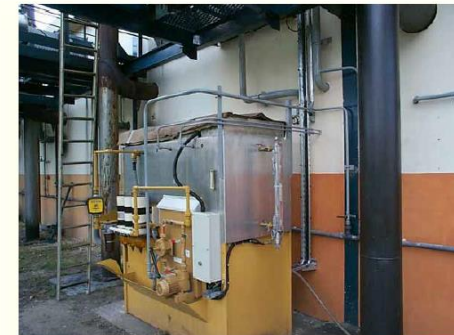
2004 GENSET. 300KVA Power Station of ENERCAL (Utility) New Caledonia
