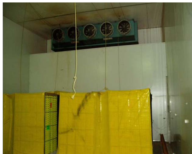
Fig 4; Air being forced through pallets by suction of fan in plenum wall
