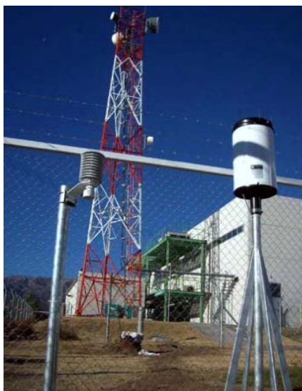
Figure 52 Meteorological Stations, installation works
