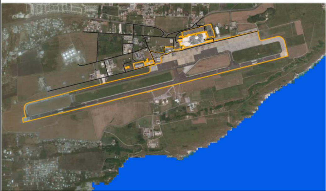
Coastal Infrastructure: Barbados, Grantley Adams airport: 2.0 m rise in sea level
