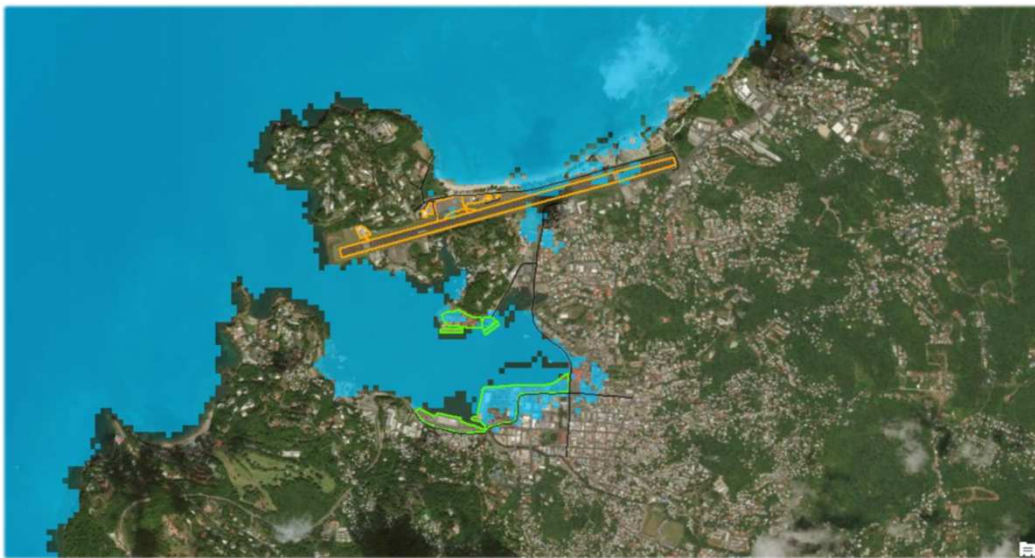
Coastal Infrastructure: St. Lucia, George F.L. Charles airport and Port of Castries: 1.0 m rise in sea level
