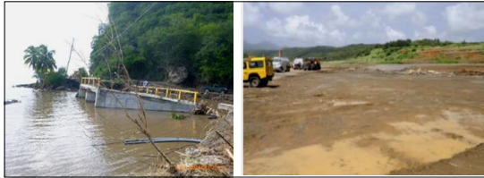
Transport infrastructure damages: (a) bridge and (b) airport apron
