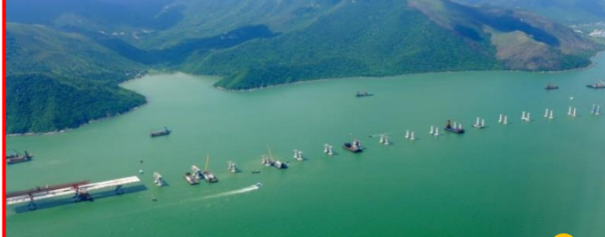
Hong Kong-Zhuhai-Macau Bridge
