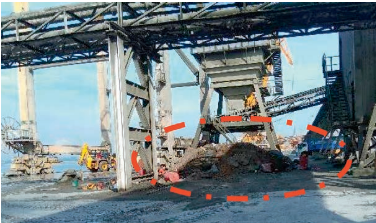
Figure 25: Accumulated waste product shown piled up under gantries in the bulk quay area
