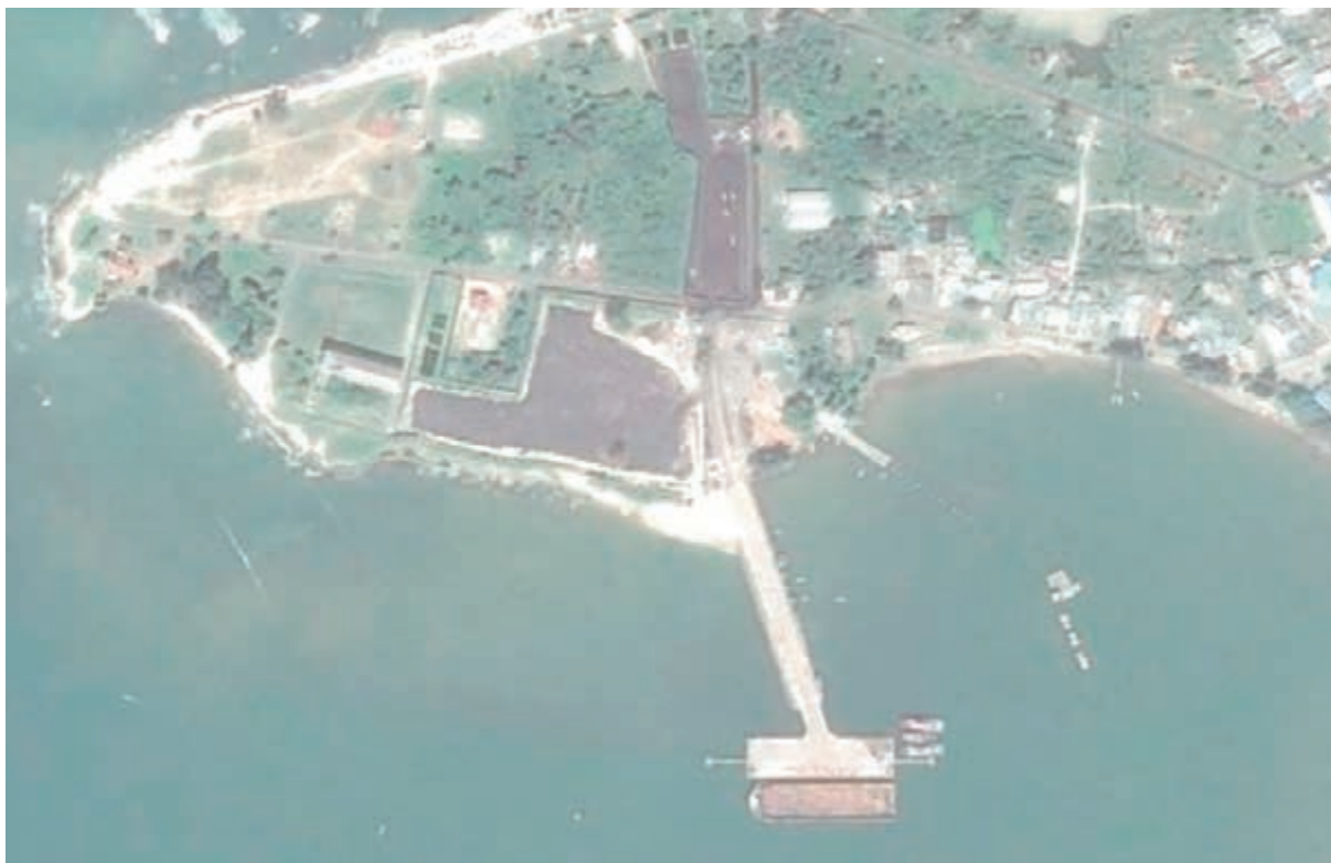
Figure 21: Aerial view of jointly operated jetty
