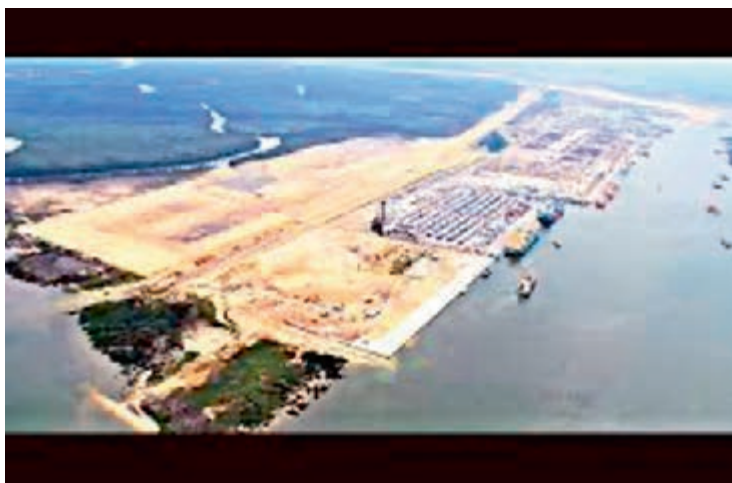
Figure 70: Onne Port on the Bonny River Channel
