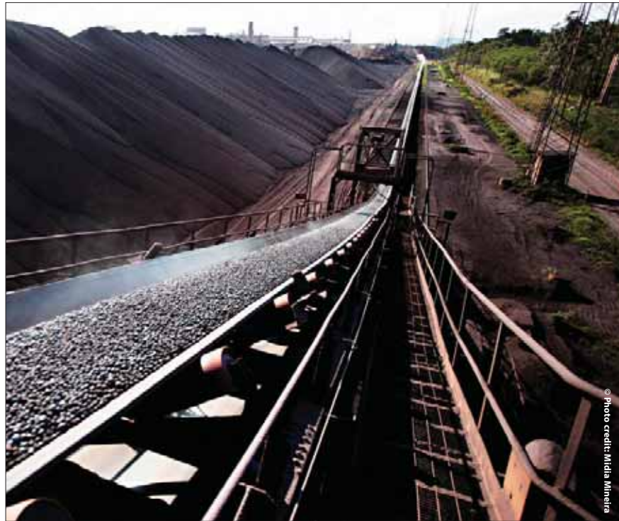
Mining operation in Minas Gerais, Brazil
