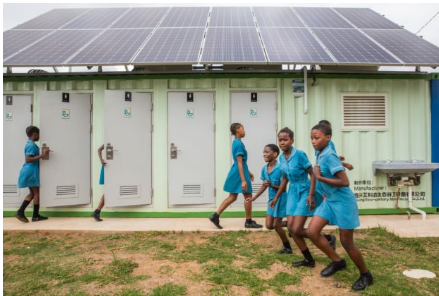
Figure 11. Water and energy saving toilets for girls in a school, Kenya
