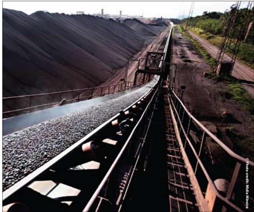
Mining operation in Minas Gerais, Brazil
