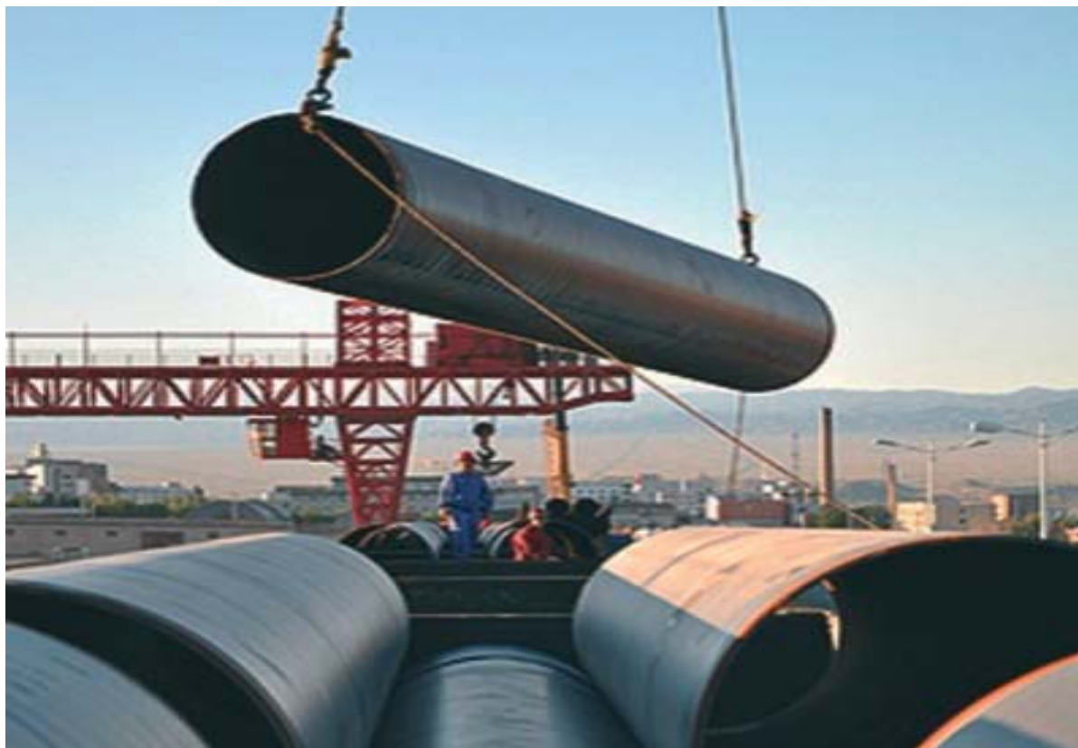
Construction of China-Central Asia Gas Pipeline
