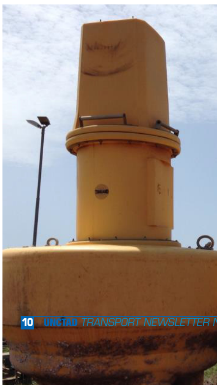
Buoy showing signs of being "sling shot" highlighting the abrasions at the top of the buoy structure
