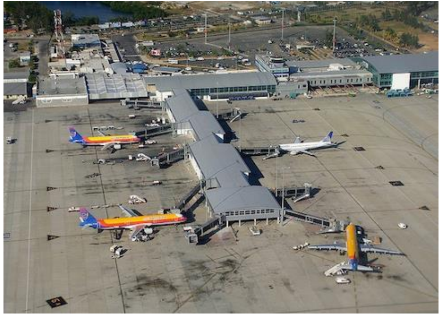
Figure 4.6 Aerial view of terminal building, control tower and gates.
