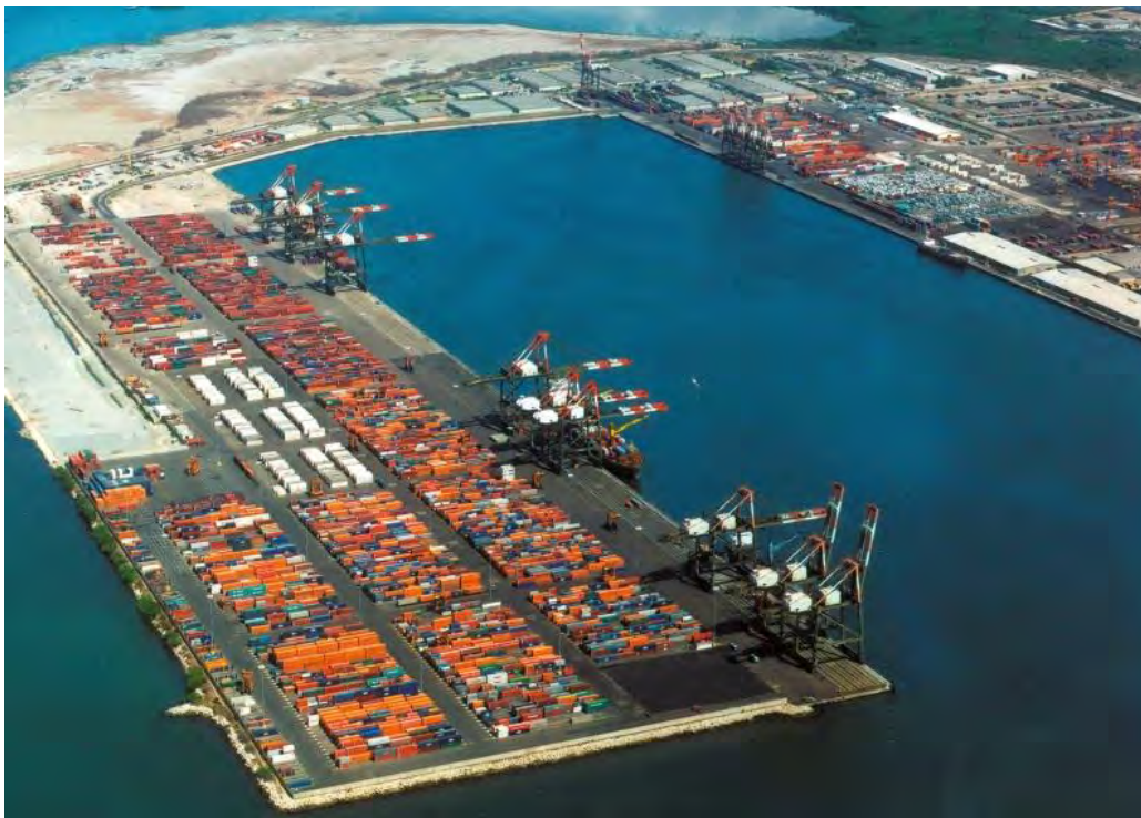
Figure 4.17 Image of KCT showing terminals, cranes and wharves.
