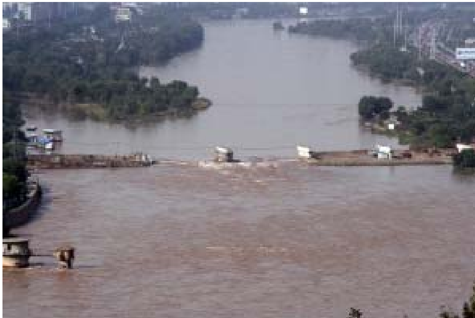
Damages of Harbor Facilities in Lanzhou, Ganxu Province in 2010
