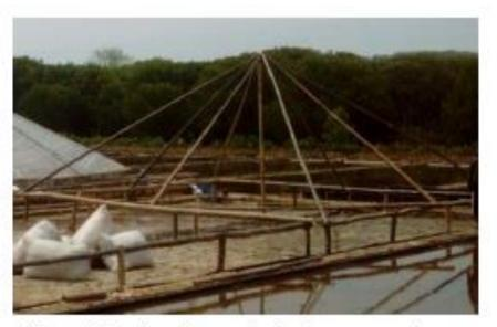
Figure 1. Bamboo framework of a low-cost greenhouse.
