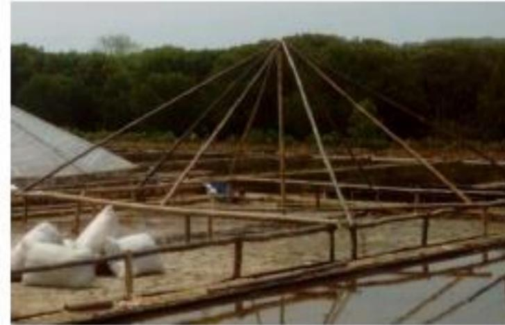
Figure 1. Bamboo framework of a low-cost greenhouse.
