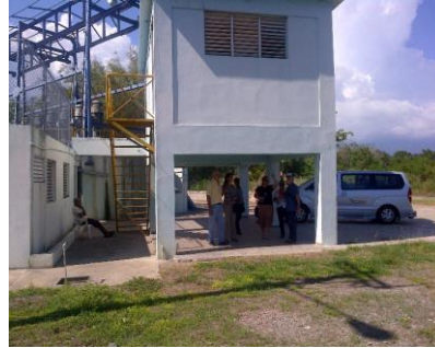
After a major flood, a pumping station in Santo Domingo was raised by the height of a person to avoid future impacts. (Source: ICF)
