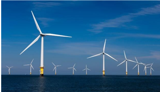
Predict.AI - Asset Health & machine performance – wind turbines & solar farms
