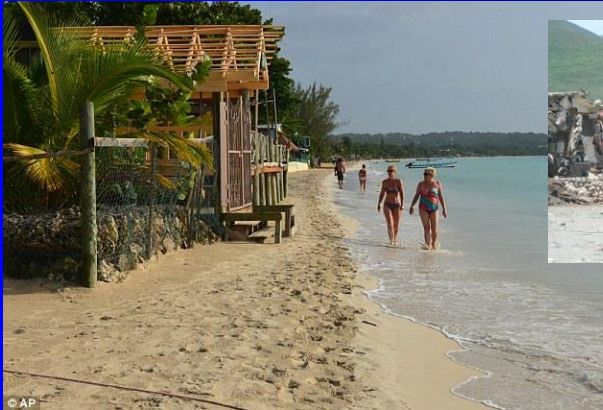
Negril, Jamaica – 1m/year erosion rate
