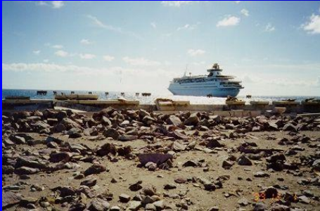
Port Zante, St. Kitts following Hurricane Lenny, 1999
