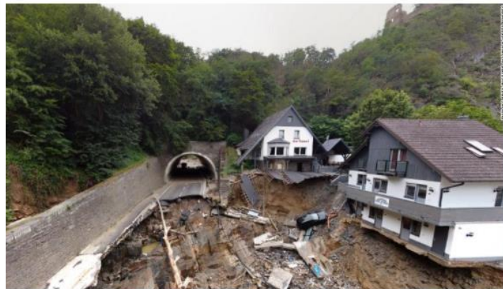
Flooding in July damaged the main road leading through the Ahr river valley in Germany.
