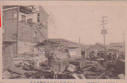
(Broken house at Tsukishima, Tokyo)
