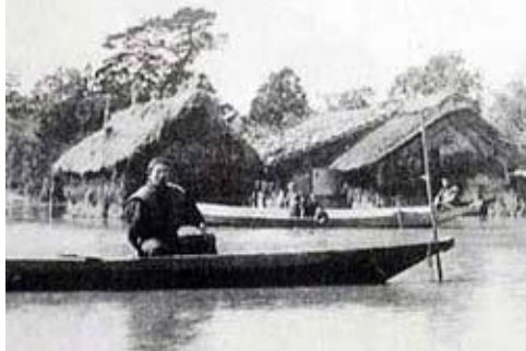
(Broken river banks at Kounan, Niigata)
