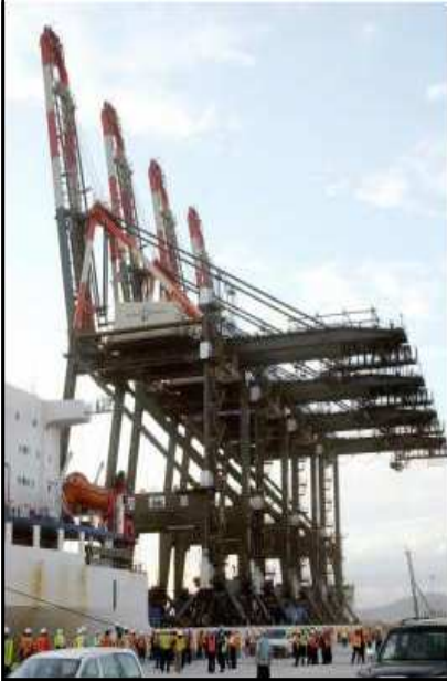
Kingston Container Terminal: Delivery of 4 Super Post-Panamax Ship-to-Shore Gantry Cranes, 2005 (Photo: Gleaner Newspaper)
