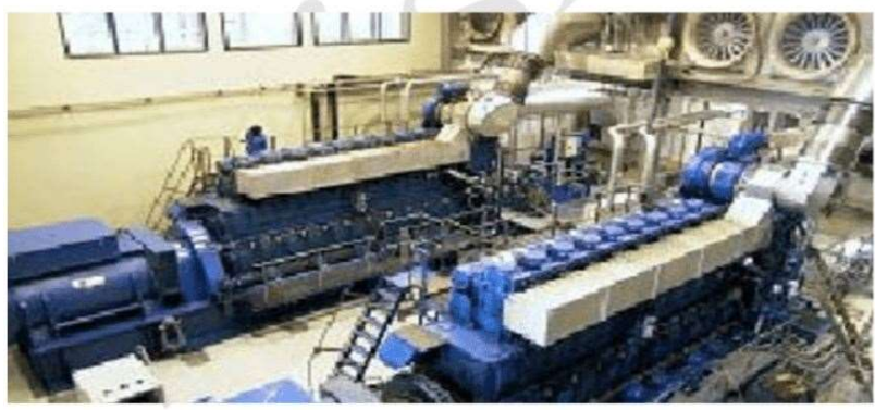
UNELCO Generators in Port Vila running on coconut oil fuelblend (Source: UNELCO).
