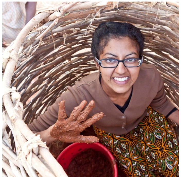
Consortium member Nadia Elkordy gets her hands dirty spreading clay inside an air-tight grain storage structure during the MIT Design Summit in Zambia. Photo: Bianca Anderson
