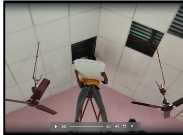
Installed polyfloss in 12 classrooms
