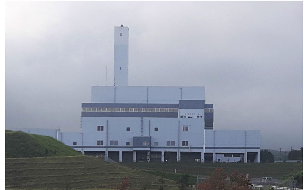
Fujisan Eco-Park Incineration Center that accommodates waste management for Gotemba and Oyama City with the capacity up to 143 ton of waste/day
