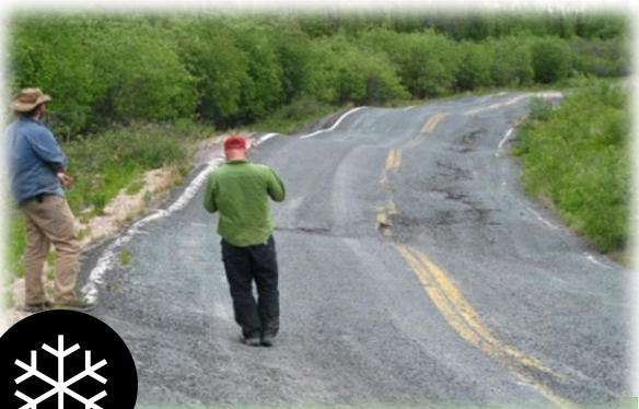
Permafrost degradation, Dempster Highway, NWT
