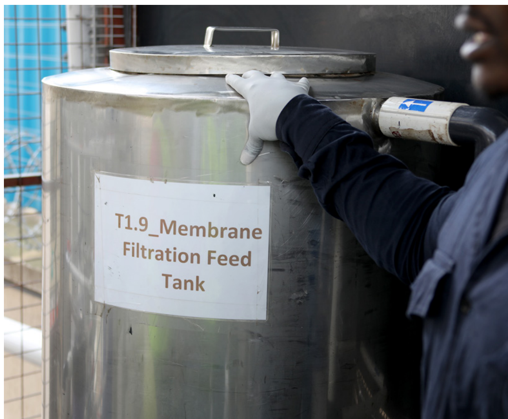
← Image 3. Membrane filtration tank at an SME wastewater treatment facility. SMEP projects in Bangladesh, Kenya, and Pakistan combine technologies such as reverse osmosis and ultrafiltration to clean industrial effluents and recover resources.
