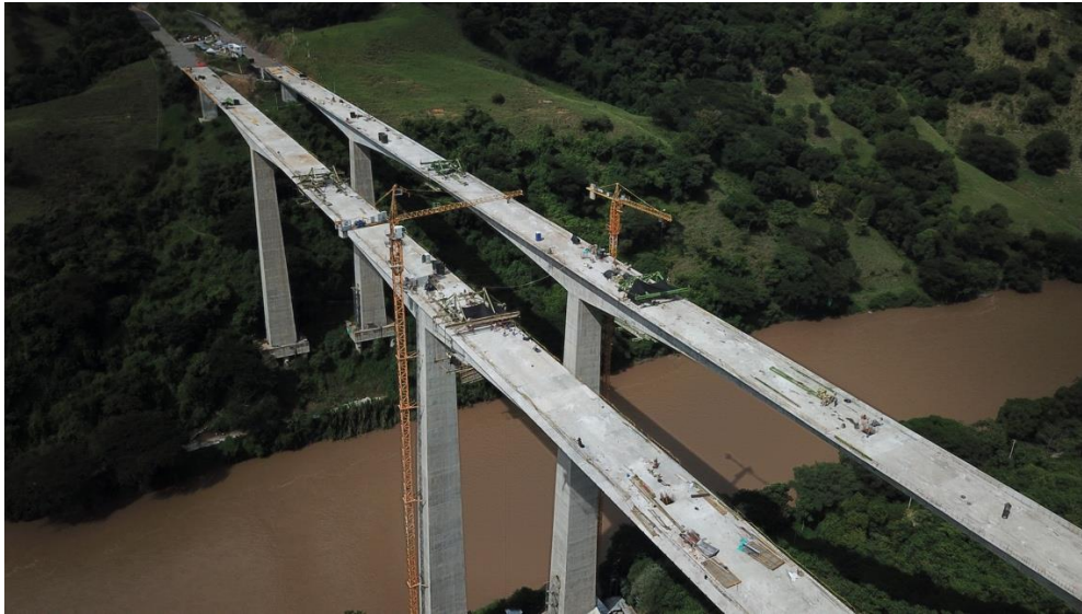
Figure 4: LC3 is already used in large-scale building and infrastructure projects. In Columbia, shopping malls and the Puente Cauca Viaduct on the Pacifico 2 road is built with LC3. Courtesy photo of Cementos Argos
