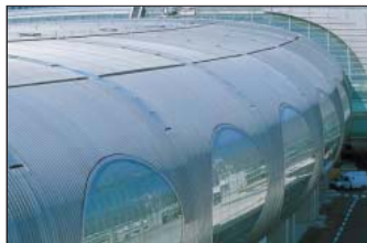
Zinc roof at an airport.
