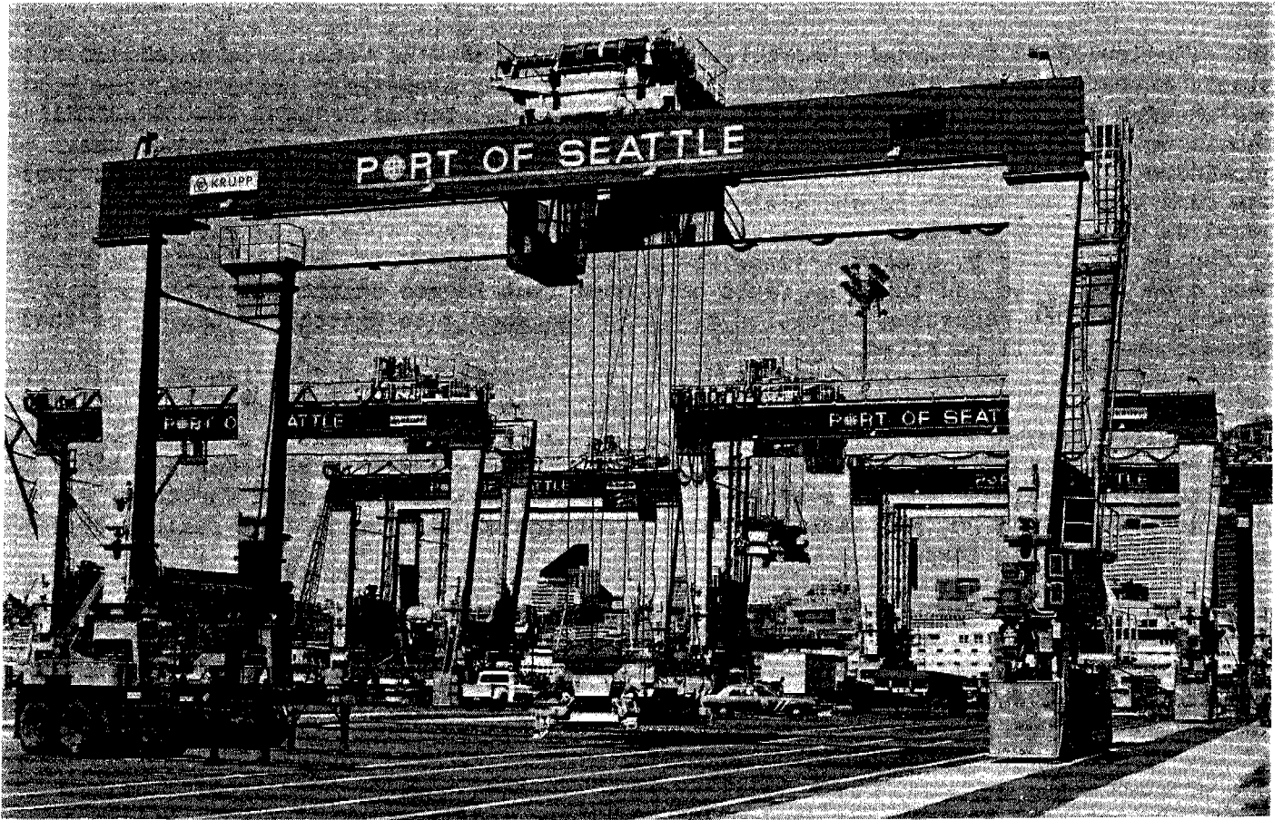
Rubber tire yard cranes being assembled
