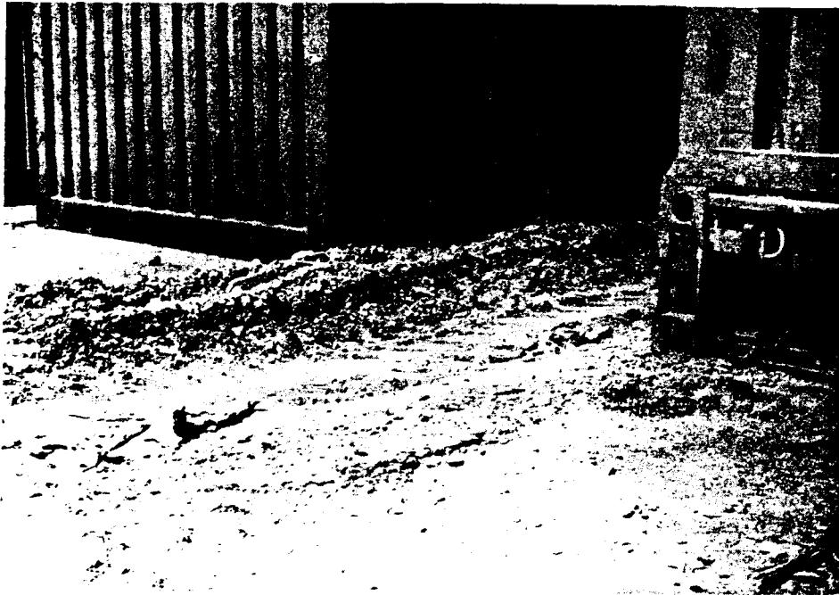
Failure of bituminous pavement in narrow aisles between container stacks resulting from channelized straddle carrier movements. The pavement was designed for the less onerous loading associated with general cargo handling.
