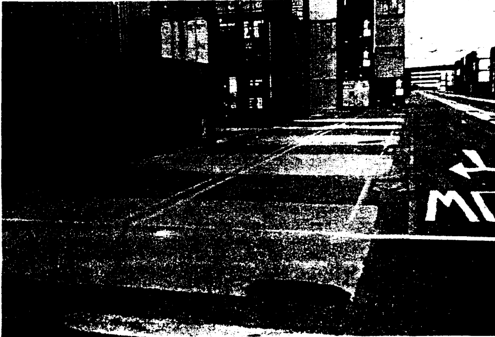
Conjunctive systems in which strips of concrete are set into asphalt so as to avoid asphalt indentation resulting from corner casting loads.
