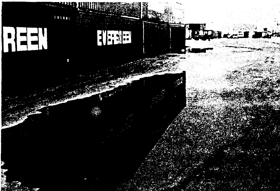
Absence of adequate falls leads to ponding.
