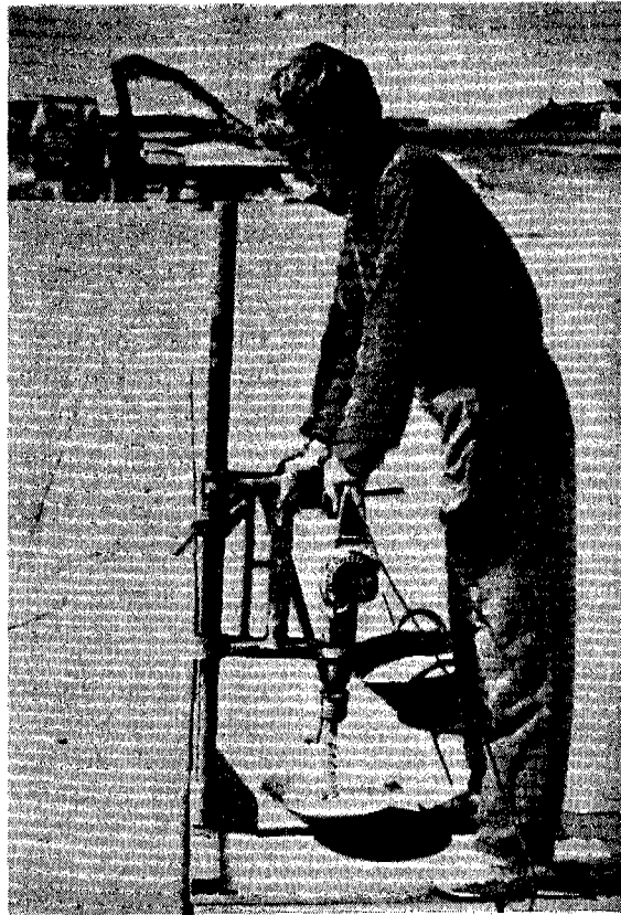
Figure 16 Vibrating roller to settle semi-rigid floating pavement
