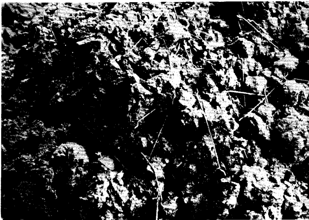
Figure 6 Concrete mix showing dispersion of steel fibres
