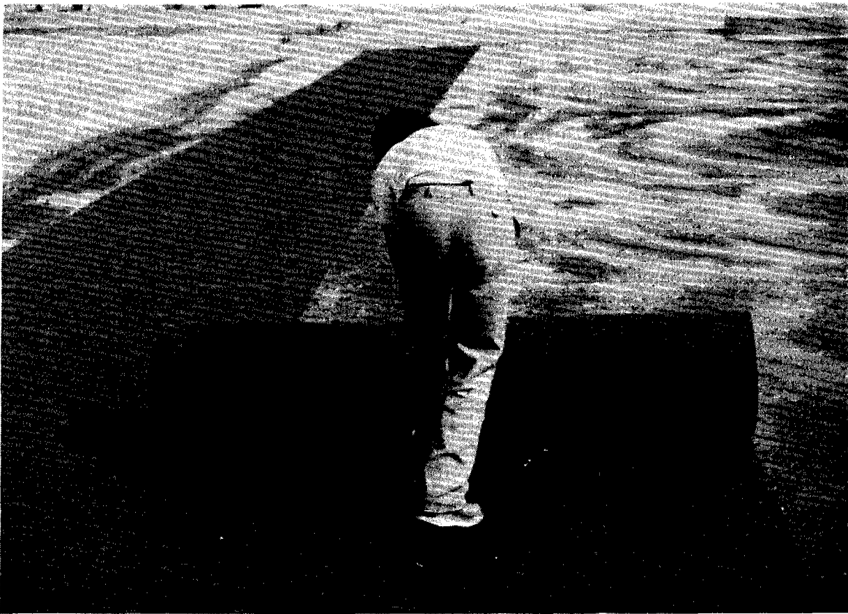
Figure 22 Application of geotextile membrane after spraying surface with tack coat
