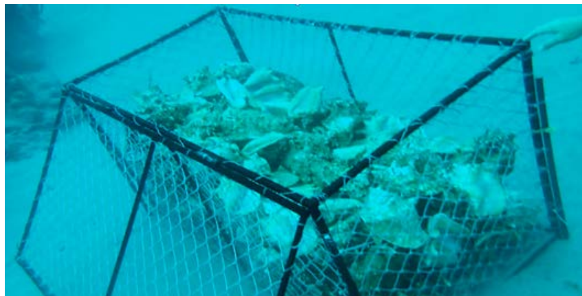
Figure 18. Conch baskets being constructed for coastal protection in Soufriere, Saint Lucia
