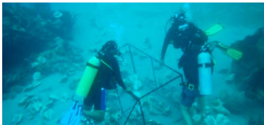
Figure 19. Conch baskets being constructed for coastal protection in Soufriere, Saint Lucia
